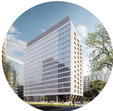
Atrium 2 Skanska Property Poland
